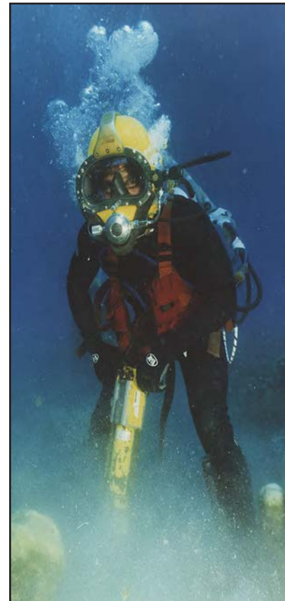
Figure 6-4. Underwater Construction Diving.
